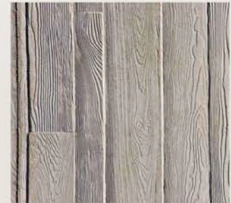
BOARD FORMED CONCRETE
