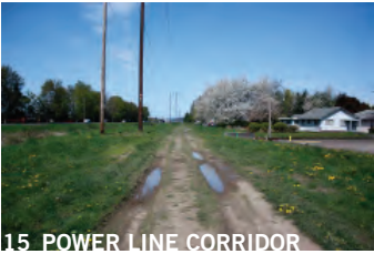
15 POWER LINE CORRIDOR
