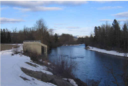
Example of a surface water intake structure
